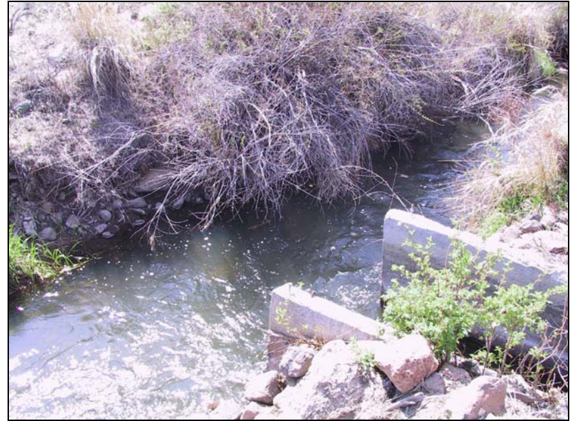
Figure 28. Diversion structure in irrigation canal.
